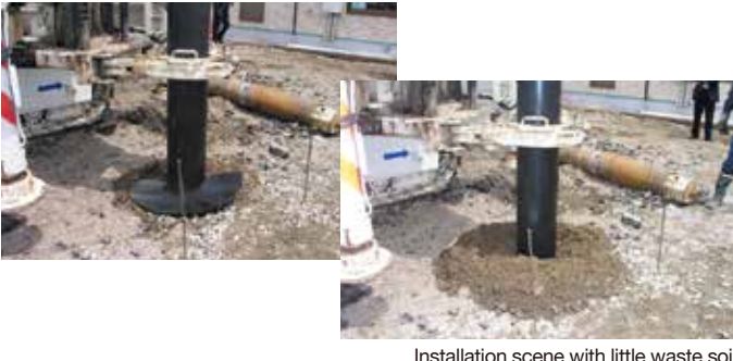
Installation scene with little waste soil
