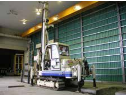
A reinforcement work for an equipment foundation inside the room (EAZET)
