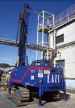
EAZET work close to the pipe rack (EAZET)
