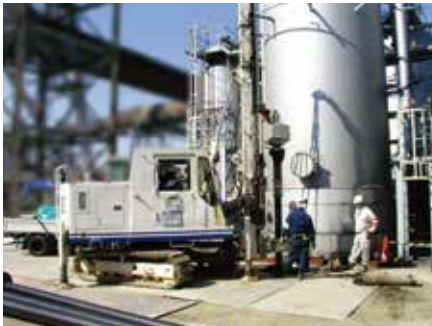
A work close to a tank (EAZET)
